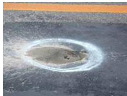
Fig. 3 Erosion on RC slab
